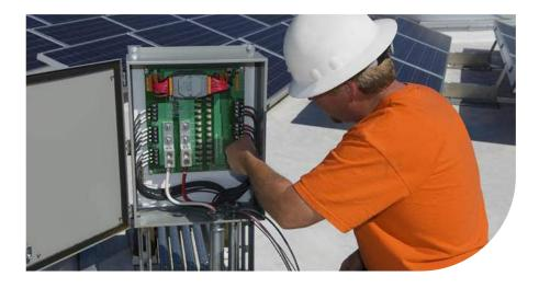
What is needed for a solar panel system: proper cable management, for starters. Panels have to stand up to all environments and endure small animals living underneath them, so correct routing, supporting and organising of your cables is key to protecting them.
